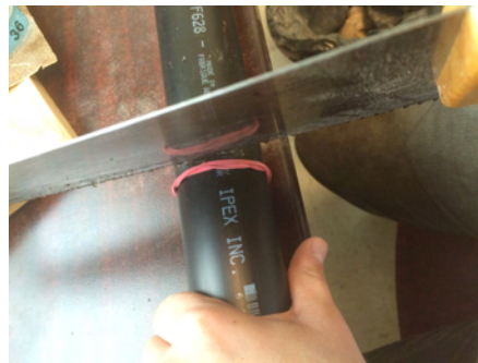
Figure 17: Step 1: Cutting the PVC pontoons.
