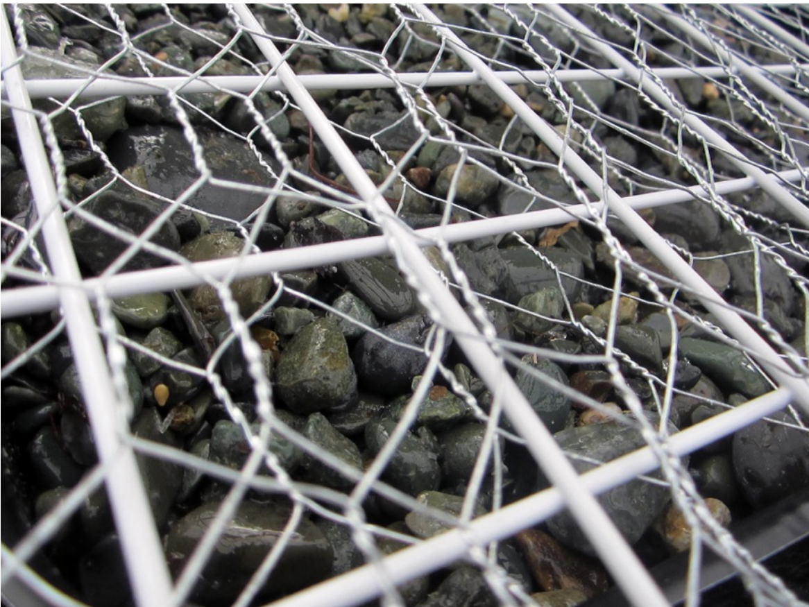
Figure 13 (below): Detail of the double mesh on the PED ROC and the rocks filled in.
